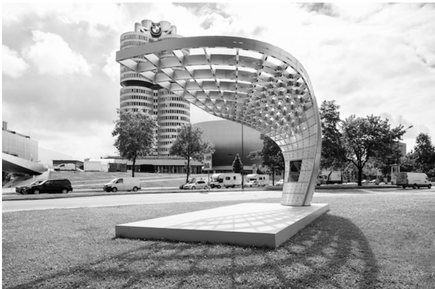
Fig. 2: point_one - solar supercharger (hand-warped plane 3 mm aluminium sheets) architecture: LAVA and designtoproduction, Stuttgart
