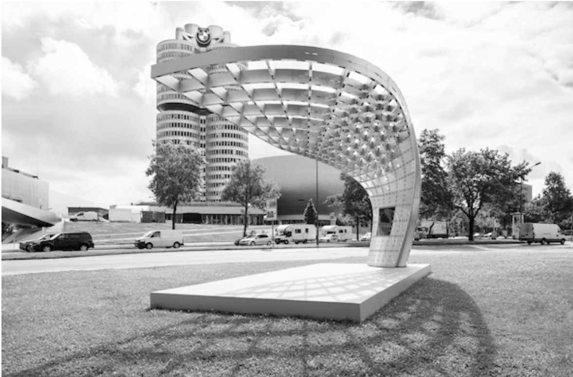
Figure 10: Point_One – the solar supercharger for BMW (hand-warped plane 3 mm aluminium sheets)
