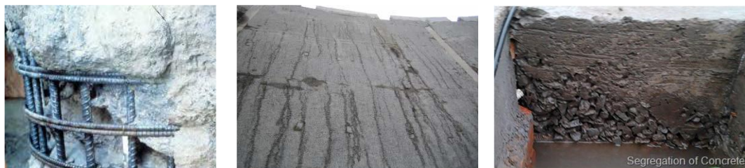
Figure 1. Construction defects related to fresh concret flow
