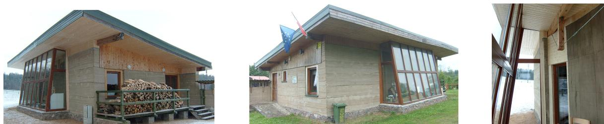
**Figure 1.** Left and in middle: View of the experimental earth building located in the Ecological Park in Pasłek. Right: The inside of the veranda. Wooden structure glazed with low-emission composite panes. On the right there is an accumulation wall made of compacted raw earth and a door connecting with the main hall.
