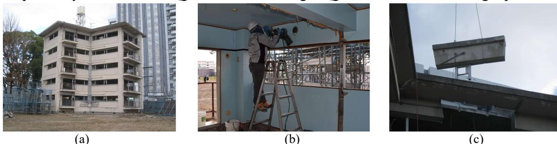
**Figure 1.** Existing building (a): comprehensive view of the test building; (b): concrete core boring; (c): cutting girder with a wire saw.
