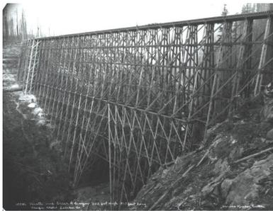
Figure 1: The Cedar River Valley logging trestle, built in 1925, used 30 metre whole timbers as primary structural elements (Courtesy of Maple Valley Historical Society).
