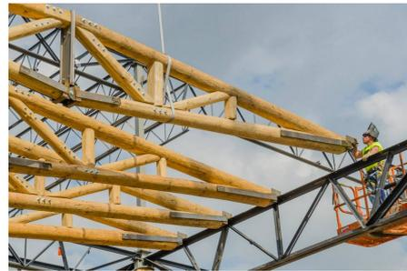
Figure 2: The Festival Foods grocery store, built in 2016, uses whole timbers from overstocked forests in 16 metre trusses (Courtesy of WholeTrees Structures).
