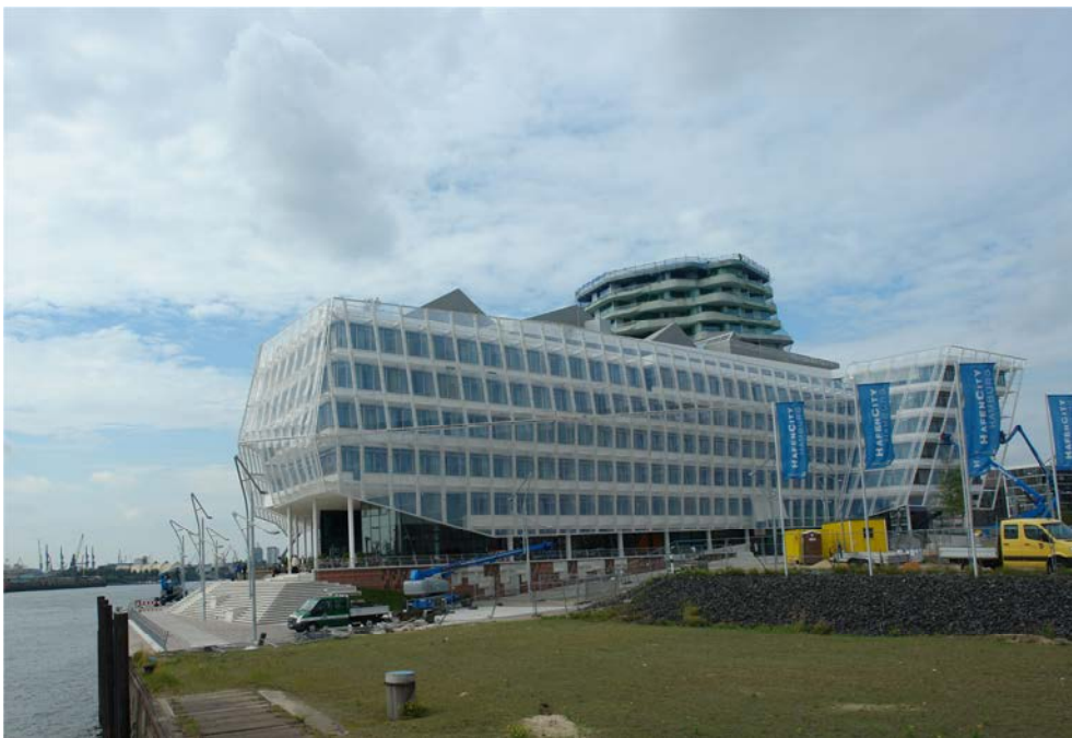
Unilever Hamburg, ETFE foil façade, picture: formTL
