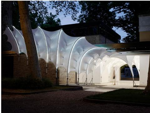
In order to steer the material behaviour of *Isoropia* we have developed a new knit structure, using a fibre (Dyneema™ by DSM), which hardly elongates under load. We assume, that the elasticity of the knit is hence only triggered on loop level. The monitoring of the behaviour of *Isoropia* focused hence on both the global structural, as well, as the behaviour on material scale.
