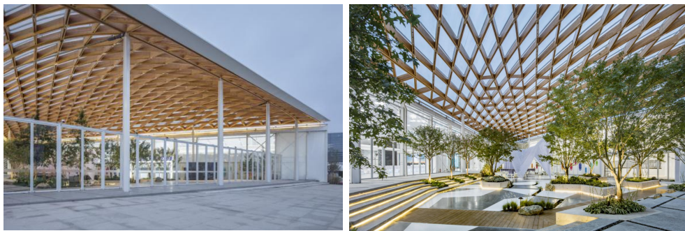
Figure1: Steel-timber gridshell of Vunue B for 2018 World AI Conference, Shanghai
