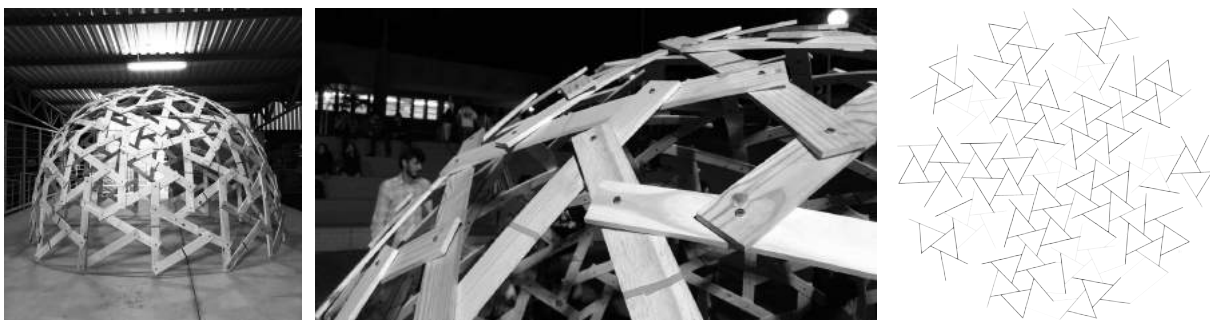
Figure 1: Prototype - reciprocal frame structure. Figure 2: Detail - coplanar joints. Figure 3. Configuration - dome topology
