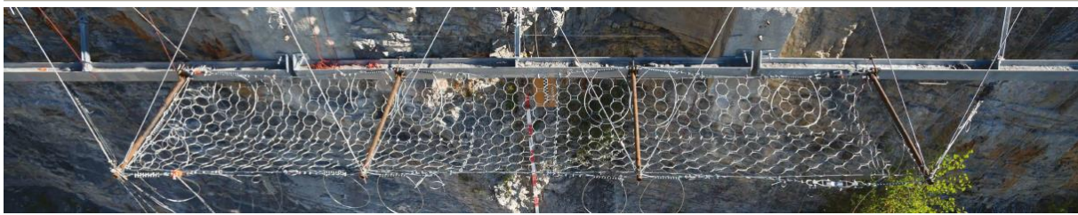
Fig. 1 C2ROP 350kJ rockfall flexible fence under study
