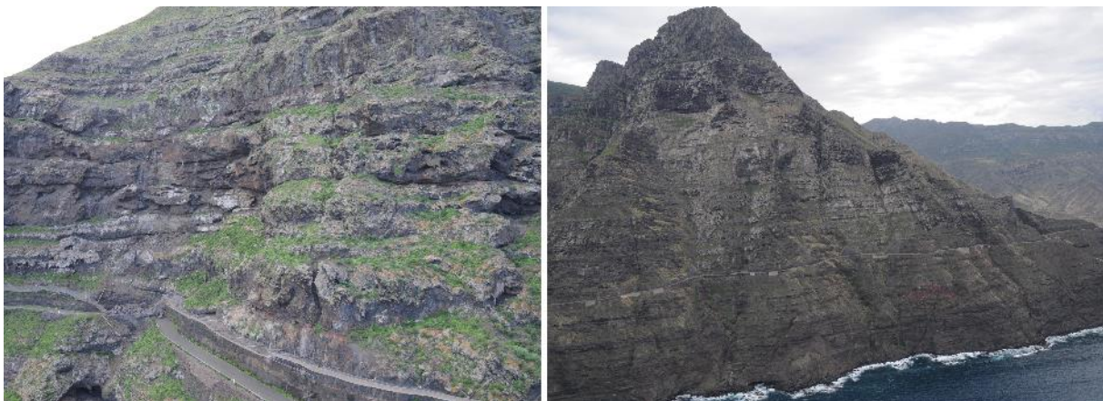
Fig. 1 The GC- 200 road between the localities of Agaete and Aldea. It is considered one of the most hazardous roads in Europe. Numerous rockfalls cut the road off every year.
