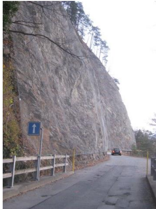
Fig 1. TECCO drapage installation in Vaduz, Switzerland-Geobrugg 2011
