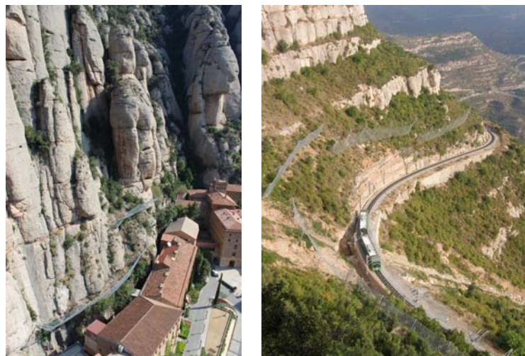
Fig. 2 Protective works for both building area and terrestrial access infrastructures.
