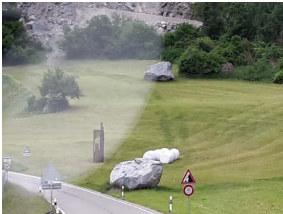
Fig. 2 Most – but not all – rocks come to a stop on the debris cone or are retained in the protection dam.
