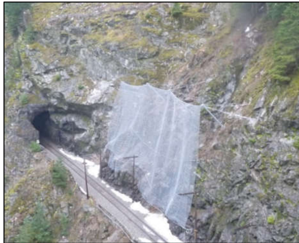
Figure 2. Attenuator installation showing series of hinged posts with support cables, and a freely hanging net.
