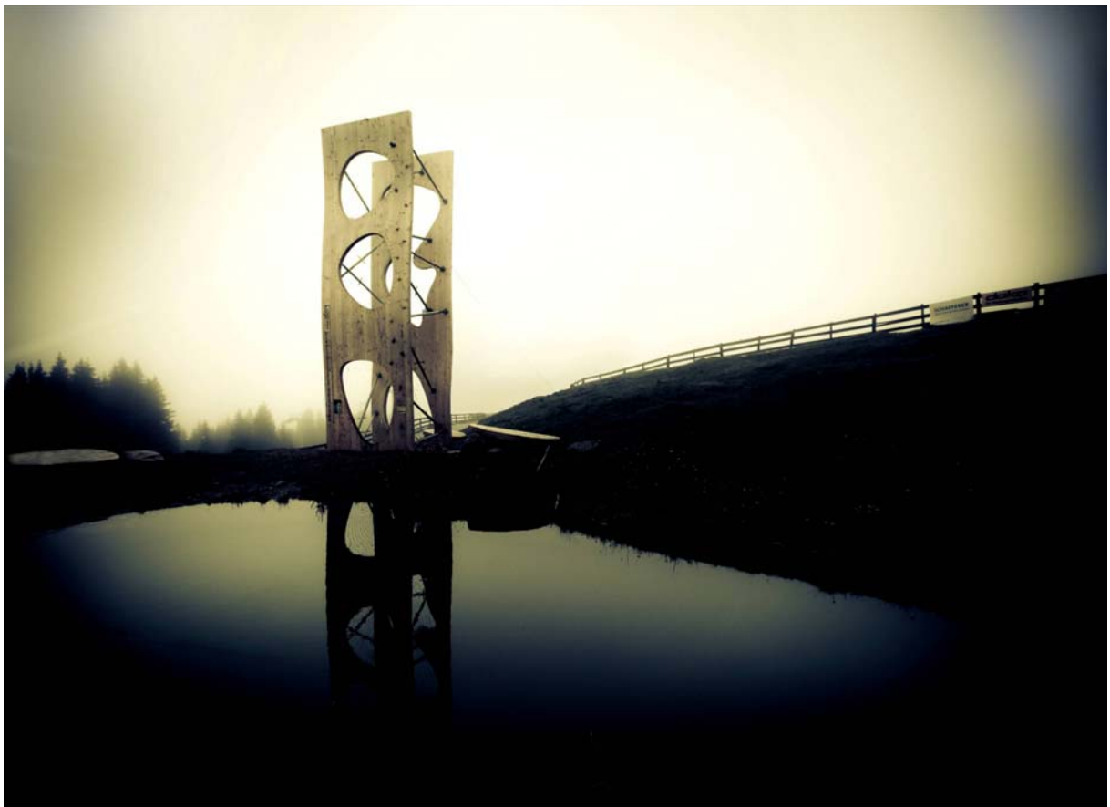
Fig. 16 "cut.enoid.tower" - impression of the finished structure on 1650m above sea level
