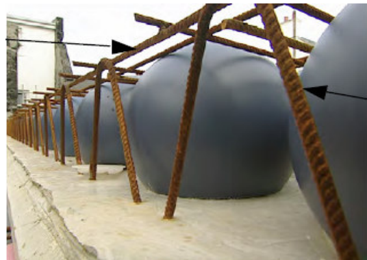
Reducing the amount of material used where less is needed is another principle used to lighten structures. Examples include the vaults used in flooring slabs and the more recent Bubble Deck technology, which uses plastic balls to lighten biaxial reinforced concrete slabs (Bubble Deck, 2006).
