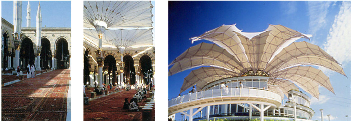
Folding structures can adapt to climatic conditions. The parasols on the Mosque in Medina (1992) and the Venezuela Pavilion at the Hanover World's Fair in 2000.
