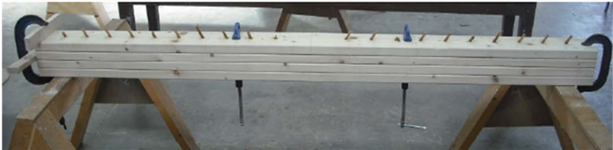
Fig. 1: Four-layer beam held in clamps during construction
