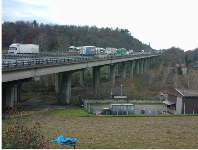
Figure 1: Bridge considered in the study.
