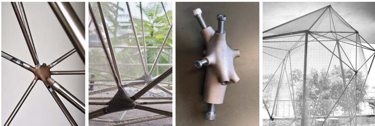
Fig 1: Images of the AIRMESH 3D Printed 1:1 prototype using bespoke metal joints, standard stainless-steel bars.
