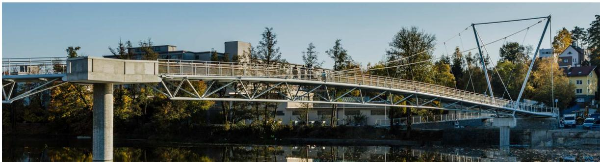
Fig.1 General outline of the asymmetric suspension span of the footbridge
