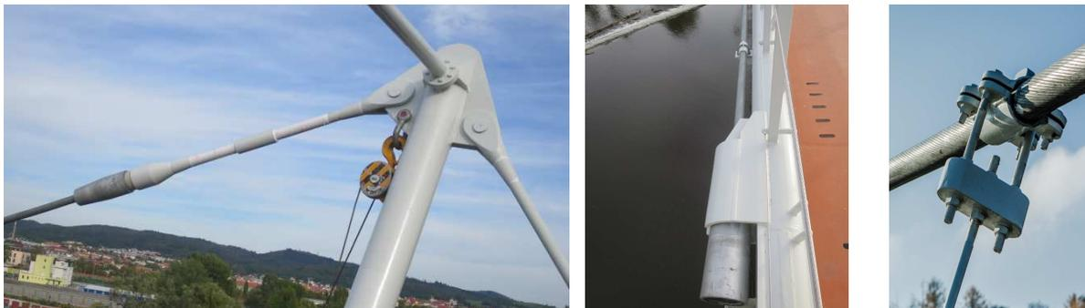
Fig.2 Structural solutions of anchoring of ropes, tendons and hangers
