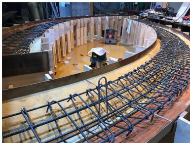
Fig.2 Construction of Precast beams
