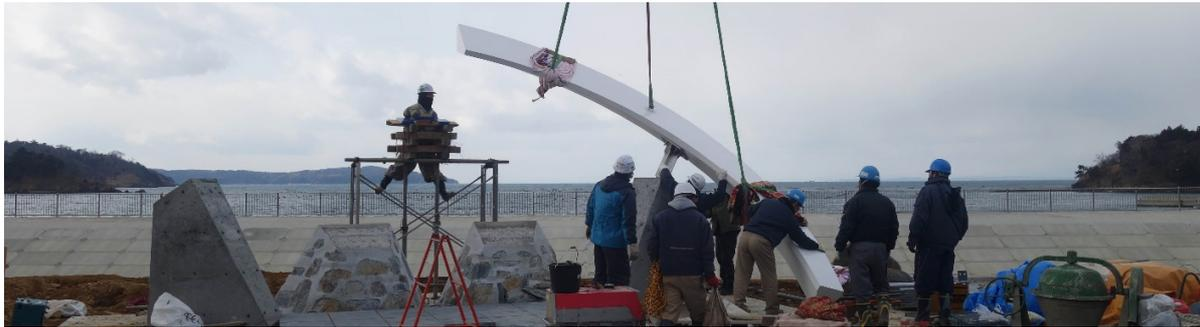
Fig.1 Precast beams set on site
