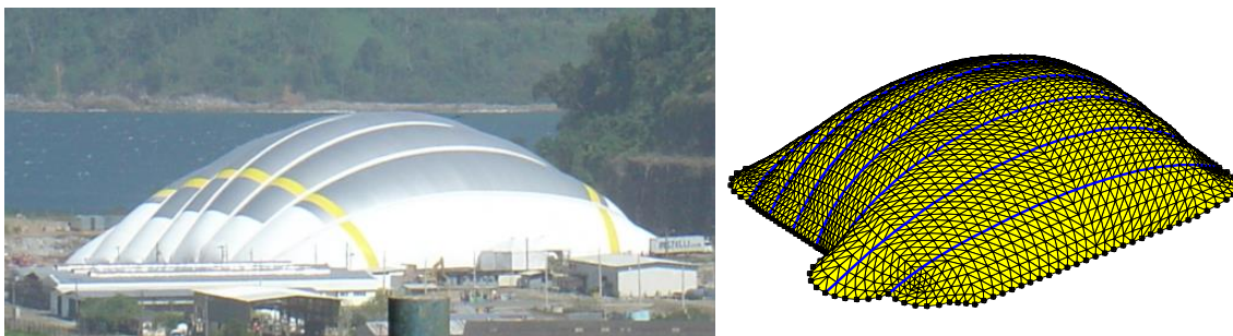
Figure 1: (a) A large pneumatic dome reinforced by sliding cables; (b) finite element mesh and equilibrium geometry under internal pressure.
