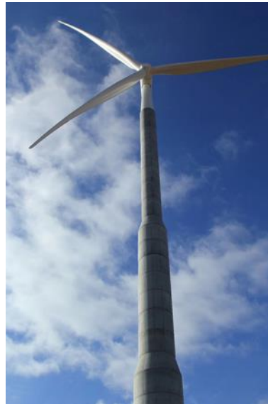
Figure 1 Photo of the concrete wind turbine tower
