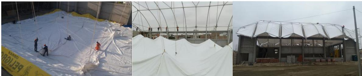
Figure 15,16,17: Membrane lifting process
