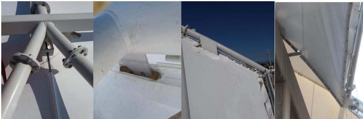
Figure 11,12,13,14: Fixation Details of membrane
