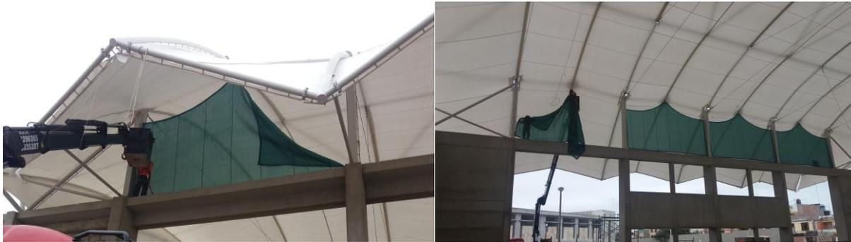
Figure 21,22: Installation of interior enclosures
