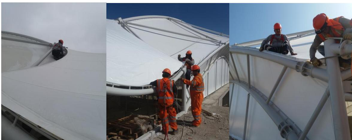
Figure 18,19,20: Installation of central module C and side module D
