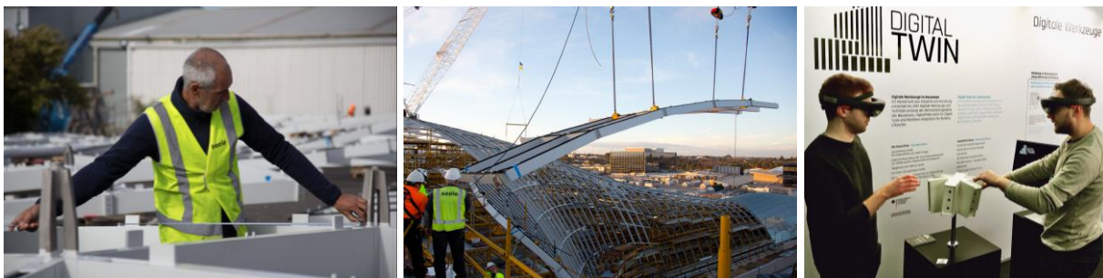
Fig. 1-2: Typical gridshell installation | Fig. 3: Demo of an AR-supported steel node installation
