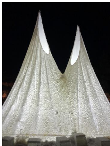
(a) TW-ICE without formwork (ext. view)
