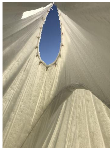
(b) TW-ICE without formwork (int. view)
