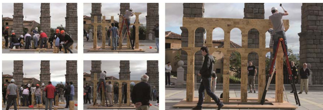
Figure 8: Construction of the aqueduct of Segovia replica
