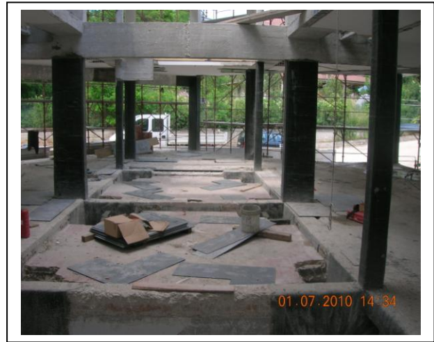
Fig.25a-25b- Concrete rehabilitation in a civil building at L'Aquila- Italy, damaged by earthquake of April 2009. Joint Column-Beam reinforcement. and Columns confinement.
