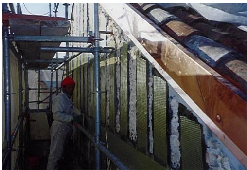
Fig. 19 -Outside walls reinforcement of Tympanum of Library .
