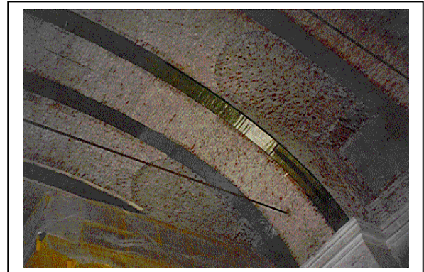
Fig. 16- Intrados reinforcement of arcades - Venaria Royal Palace –Turin. (1999)
