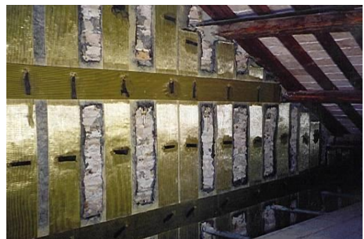
Fig. 20 -Inside walls reinforcement of Tympanum of Library.
