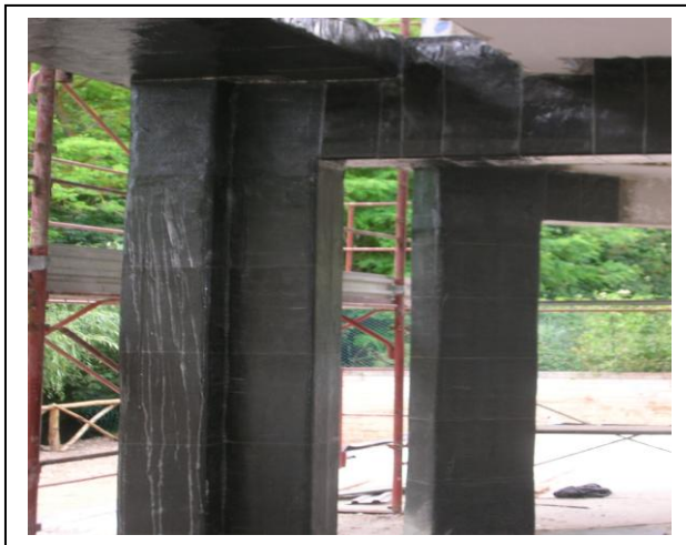
Fig.25a-25b- Concrete rehabilitation in a civil building at L'Aquila- Italy, damaged by earthquake of April 2009. Joint Column-Beam reinforcement. and Columns confinement.
