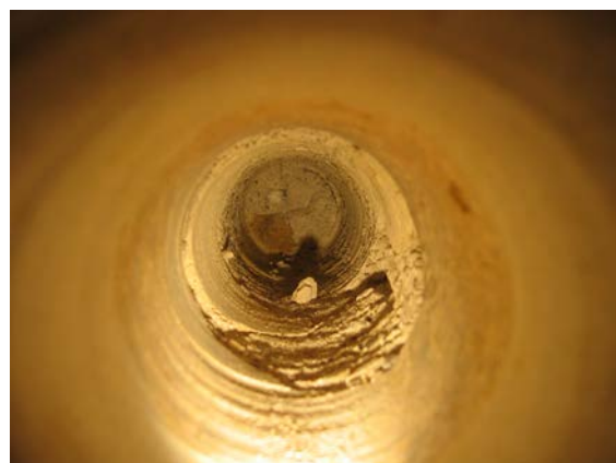
Figure-6: Inside the drill cutting
