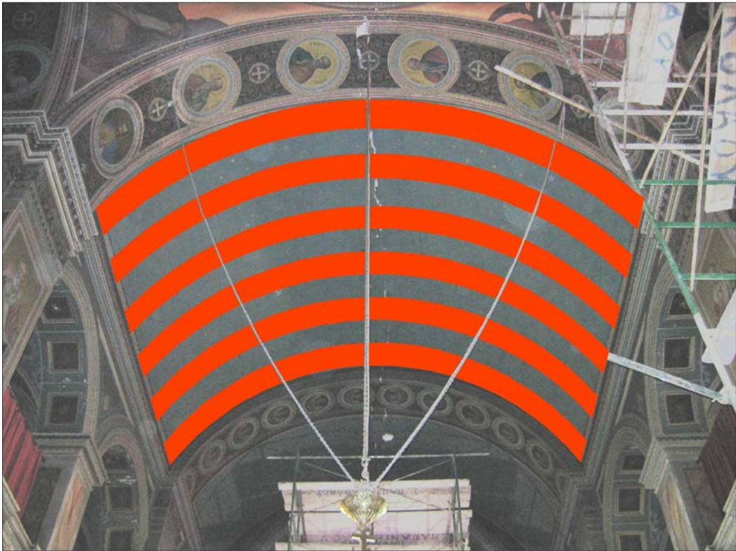
Figure-15: Placement of CFRP on the intrados of the arced ceiling
