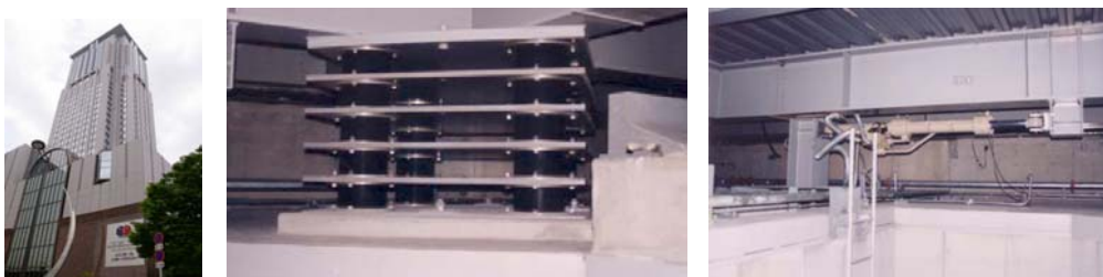
Figure 1 – a) Overview of the “Applause Tower”; b) Support equipment of the platform; c) Hydraulic actuators
