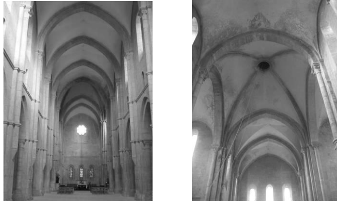
Figure 2. The vaulted system of the Fossanova church.
