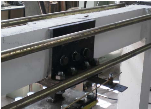
Figure 19: Concrete cover failure (F2)
