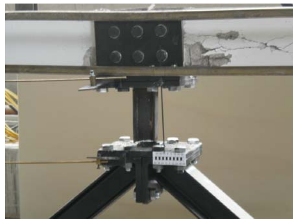
Figure 20: Cracks at the middle of the top beam (F3)
