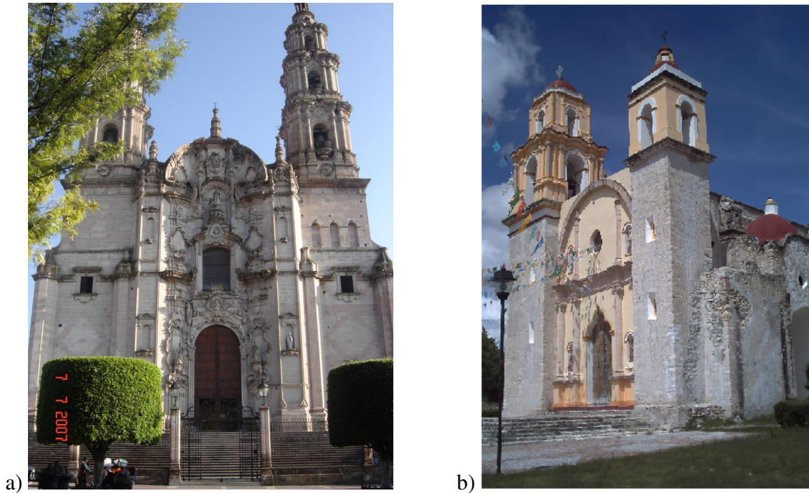
Figure 1: Typical colonial churches built in: a) low seismic risk zone (central Mexico), b) high seismic risk zone (Pacific coast).
