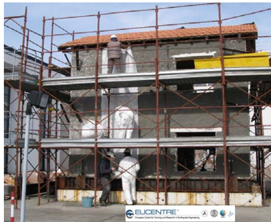
Figure 9: Masonry building with textile application
