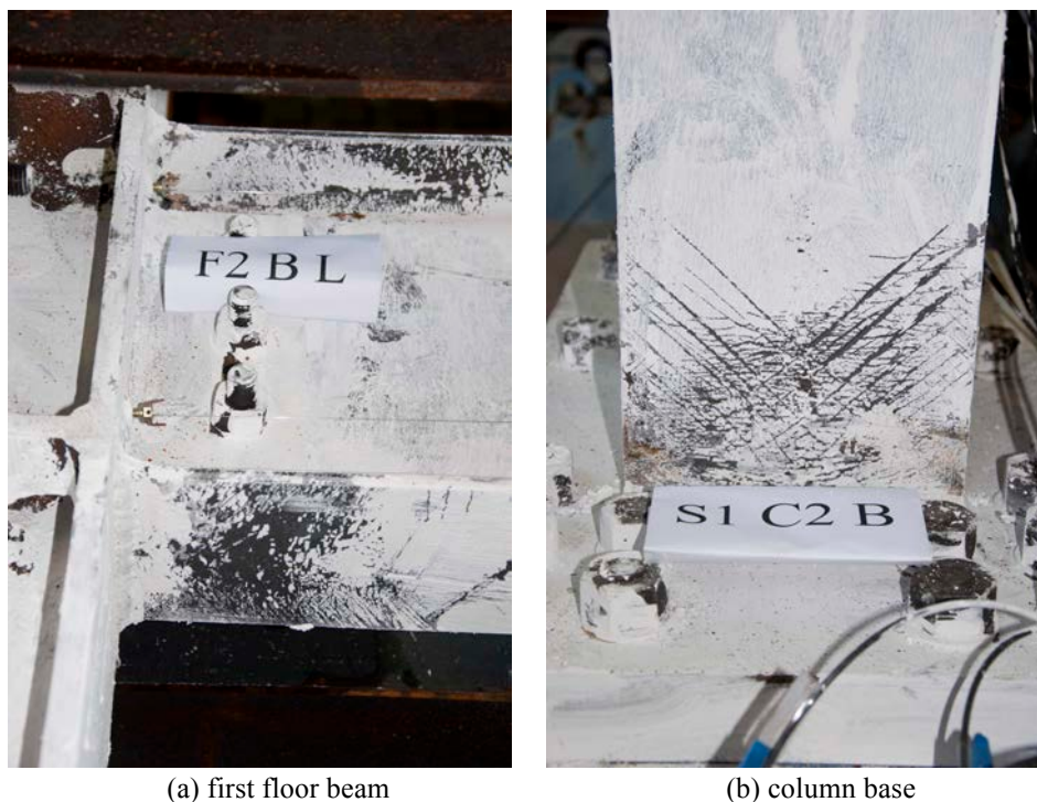
Figure 13: Structural damage observations during testing Phase I.
