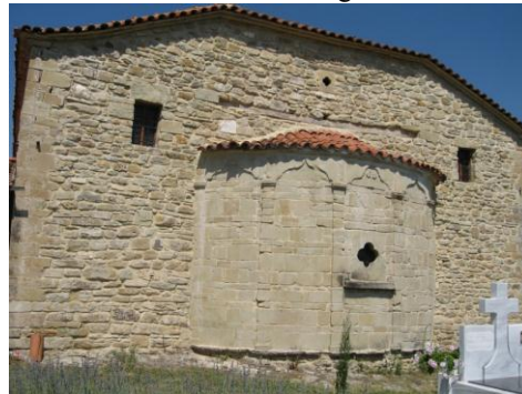
Figure 1c. East wall and Apse.
