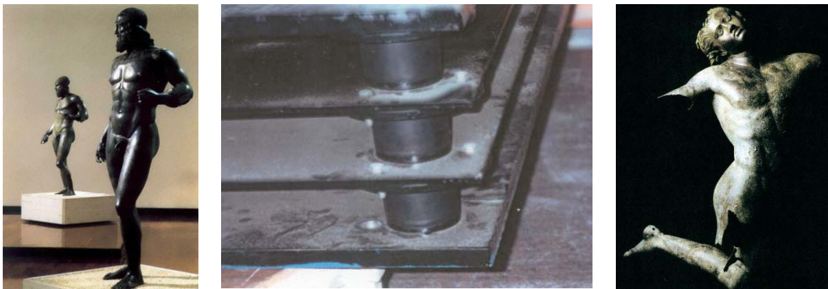
Figure 31: Bronzes of Riace , which were isolated in the Reggio Calabria Museum (seismic zone 1) in the years '90s (left); its present 3-stage HDRBs system (at the centre), which should be soon replaced by an improved SI system; Dancing Satyr in the Mazara del Vallo Museum, again protected by a 3-stage HDRBs system (right).
