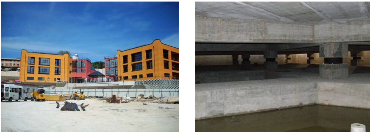
Figure 5: The new Francesco Jovine primary school and the “ Tre Torri ” multifunctional complex in San Giuliano di Puglia (now seismic zone 2), supported by a common isolated artificial ground slab, which was certified as safe by A. Martelli in September 2008 (left); their SI system, formed by 61 HDRBs and 12 SDs donated by the Italian manufacturers, during construction (right). These buildings will be seismically monitored [10, 11].
