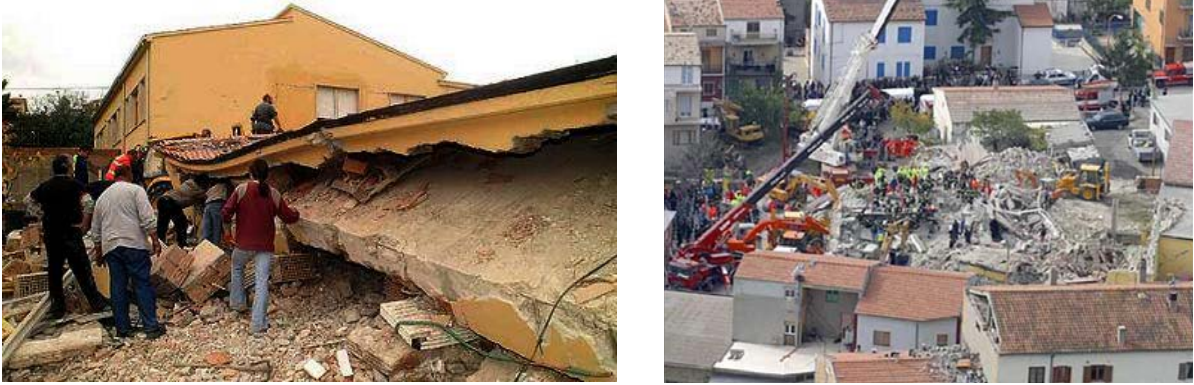
Figure 2: Collapse of the Francesco Jovine primary school of San Giuliano di Puglia (Campobasso) during the 2002 Molise & Puglia earthquake and search of survivors amid the debris. Prior to the aforesaid earthquake the San Giuliano di Puglia area was not seismically classified (now it is classified in seismic zone 2).
