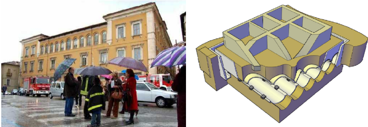
Figure 37: The De Amicis primary school in L’Aquila, damaged by the 2009 Abruzzo earthquake (left); sketch of the new sub-foundation technique patented by ENEA and the Polytechnic of Torino in 2010 (right).
