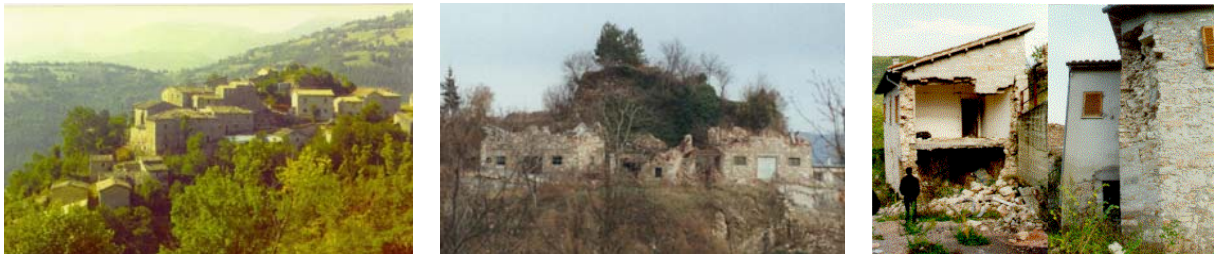
Figure 28: Mevale di Visso as reconstructed with conventional techniques after the damages suffered during the 1979 Valnerina earthquake (left) and again heavily damaged after the 1997-98 Marche & Umbria event (at the centre and right)
