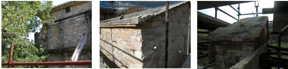
Figure 25: The Santa Croce della Ficarella Church in Case Basse (Perugia) put in safe conditions after the 1997-98 Marche & Umbria earthquake (left) and subsequent conventional restoration works (at the centre and right), which should have been followed by the construction of a sub-foundation and insertion there of a SI system formed by 8 HDRBs with 600 mm diameters and 294 mm height (maximum design displacement = 256 mm).
