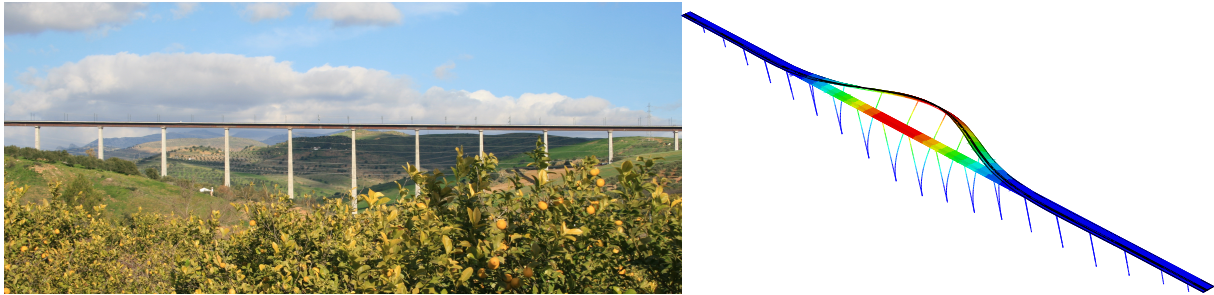
Figure 1: Viaducto “Arroyo las Piedras” in Córdoba–Málaga HS line: first mode of vibration 0.313 Hz
