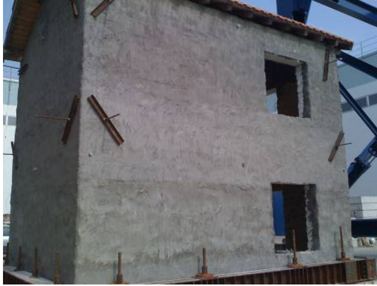
Figure 6: View of the reinforced building
