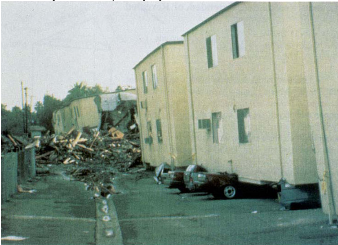
Figure 1. Loma Prieta, soft story collapse.
