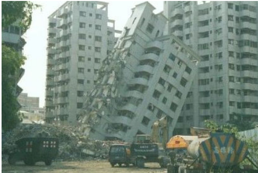
Figure 2 Taipei Structure overturning.
