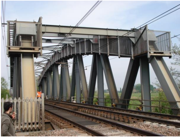
Figure 6: General view of Panaro bridge
