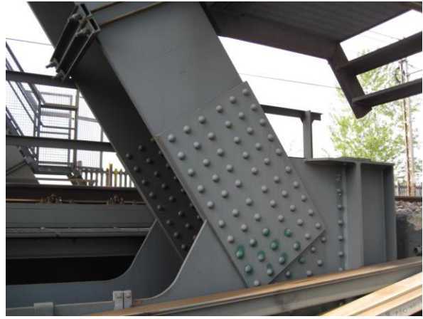
Figure 7: Riveted diagonal-lower string joint of Panaro bridge
