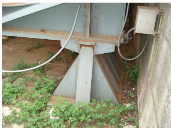
Figure 11: General view of fixed bearing
