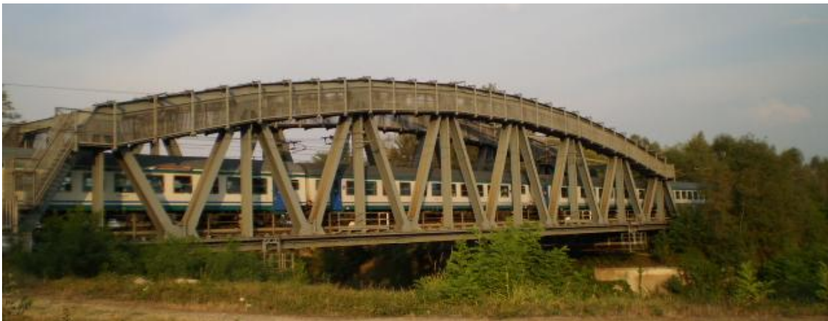
Figure 4: Picture of Panaro bridge (Courtesy of RFI).
