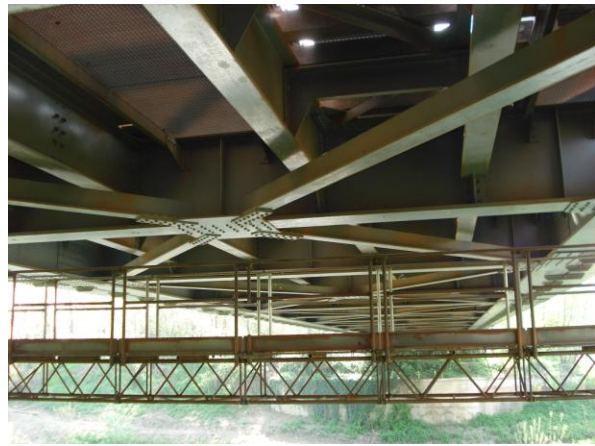
Figure 9: General view of lower and track bracings
