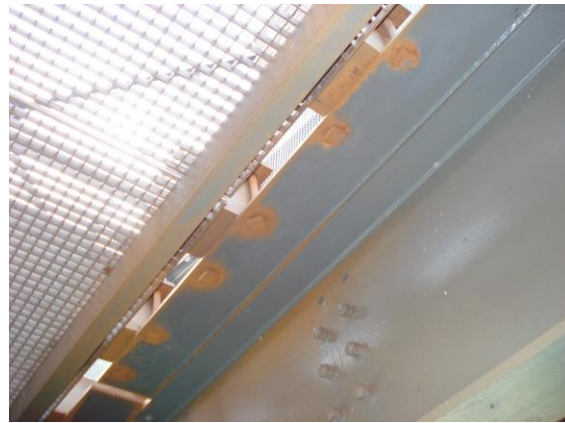
Figure 13: Sleepers-longitudinal girder connection by catch bolts
