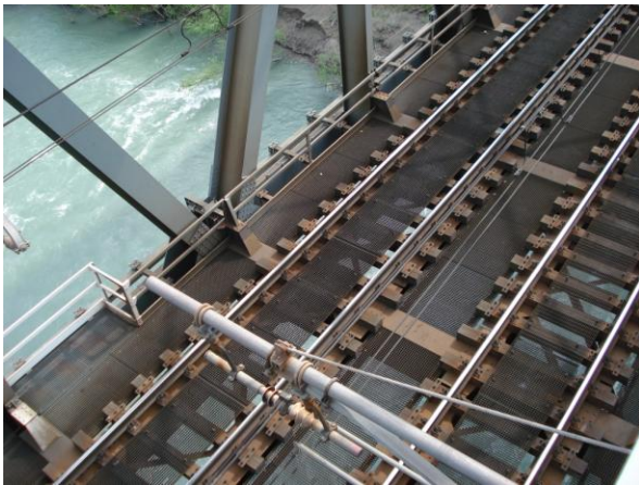
Figure 8: General view of deck structure
