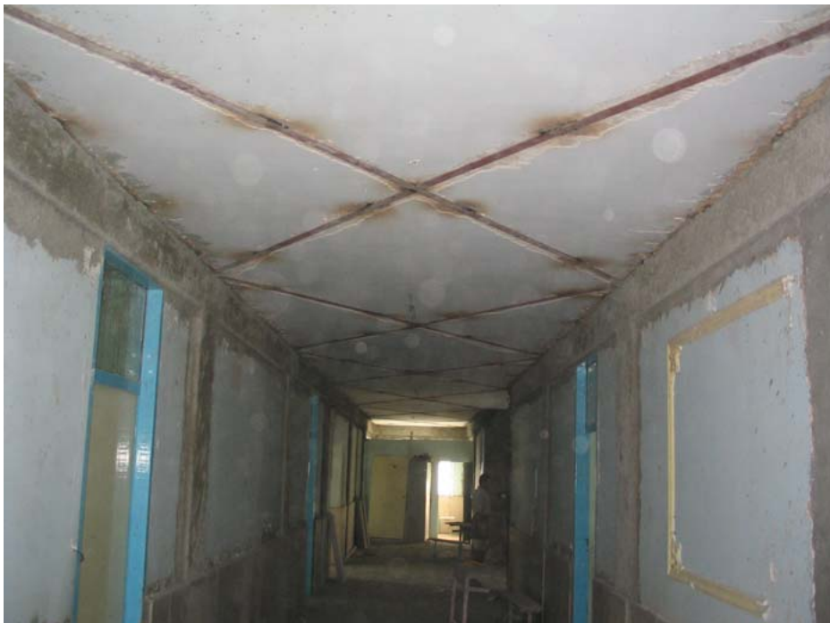
Figure 4. Adding 50 \times 5\text{mm} steel plates in order to integrate the traditional jack arch slab joists.
