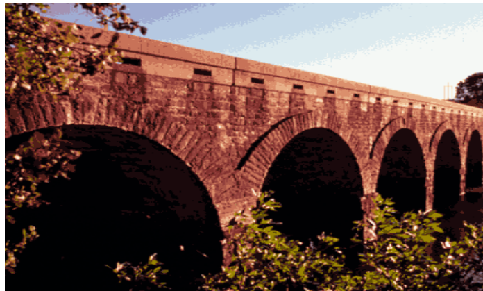
Figure 3: Masonry Arch Bridge under Study
