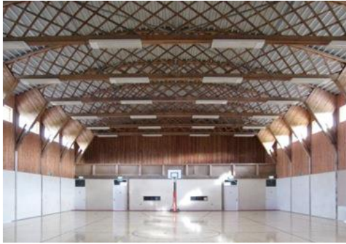
Figure 13 Wynstone School, Belfast trusses (photo courtesy of David Gregory architects)
