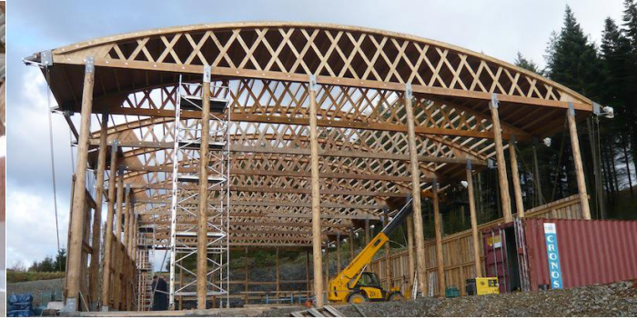
Figure 14 Belfast trusses at Esgair Timber (photo courtesy of Barratt Associates)
