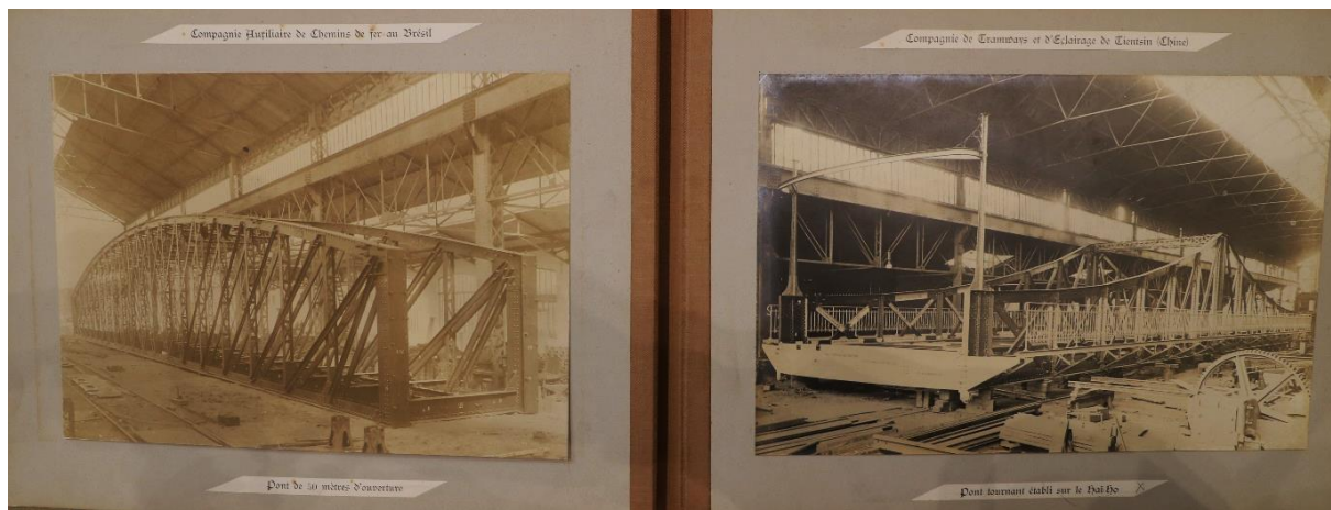
Figure 1: The company catalogue of the Belgian workplace 'La Brugeoise' depicts assembled bridges ready to be exported to Brazil (left) and China (right) [City Archives of Bruges]
