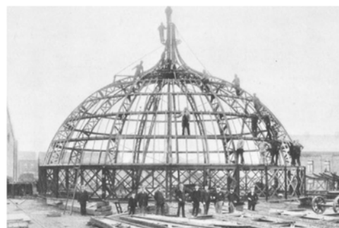
Figure 1: a) Amazonas Theater in construction [1,2]; b) Amazonas Theater steel dome in 1885 [3].
