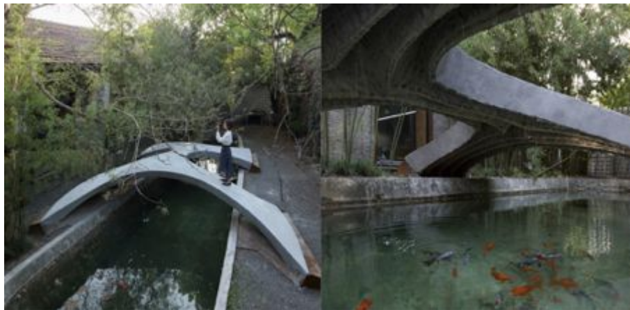
Figure 1 Images of completed bridge
