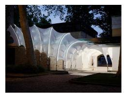
In order to steer the material behaviour of Isoropia we have developed a new knit structure, using a fibre (Dyneema<sup>TM</sup> by DSM), which hardly elongates under load. We assume, that the elasticity of the knit is hence only triggered on loop level. The monitoring of the behaviour of Isoropia focused hence on both the global structural, as well, as the behaviour on material scale.
