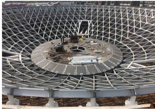
Figure 1: Inverted aluminum alloy single-layer dome in Shanghai Planetarium
