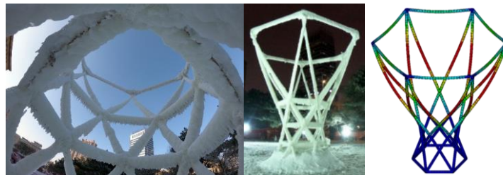
Figure 1: The world's first sprayed net ice hyperboloid structure
