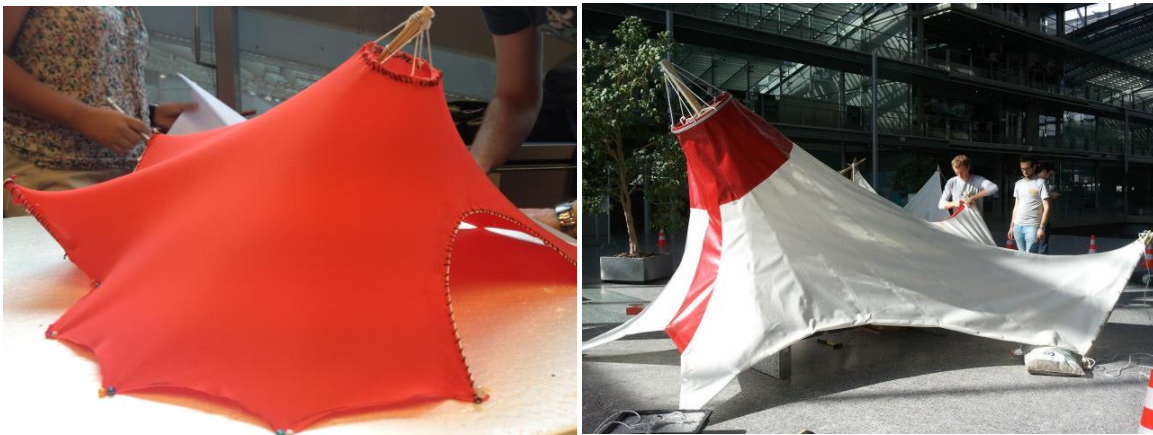
Figure 3: “El paraíso de la siesta”: Lycra model and final structure (photo by courtesy C. Douthe)
