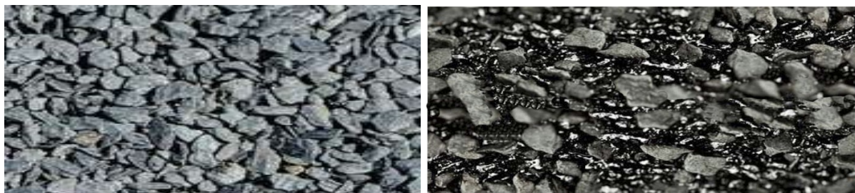
Figure 1. This is a comparison of topping on new roofing paper and topping on the same roofing paper after several years of use in adverse conditions (on the right photo a drastic example of a significant loss of granules and exposure of asphalt in a roof depression - a periodic puddle).
