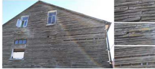
Figure 1. Case study that exemplifies the end of the service life of timber claddings.
